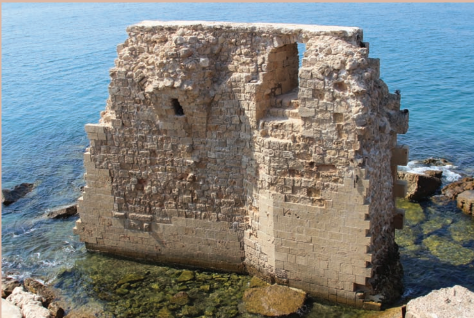
FIG. 9 Pisan Harbor wall after the completion of conservation work to protect the deteriorating stones. (Photo by J. Munro.)
