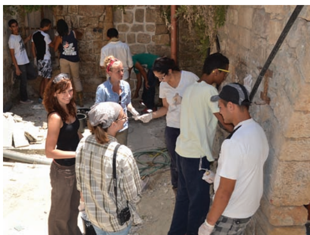
FIG. 23 Program participants applying lime mortar (pointing) to the exterior courtyard walls of the ICC. (Photo courtesy of SHARE.)
