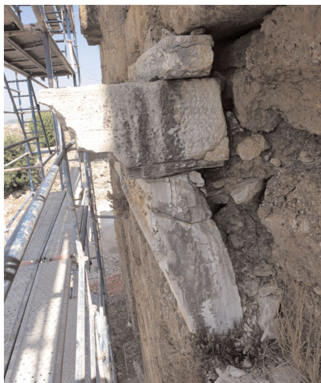
A decorated architrave frieze block, revealing the limestone block on top of the cornice as well as the row of limestone blocks below the architrave (forefront of photo). The mortared rubble connecting the decorated building elements and the conglomerate back wall is also clearly visible
