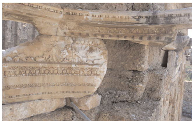
The entablature of the central niche, revealing the row of undecorated limestone blocks wedged in underneath the entablature and the conglomerate ashlars of the back wall partially cut back to receive the entablature
