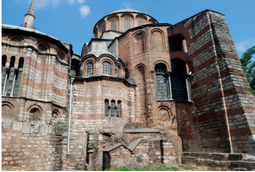
Fig. 3.9: Istanbul. Kariye Camii, view from east, showing multiple phases of construction (author).
