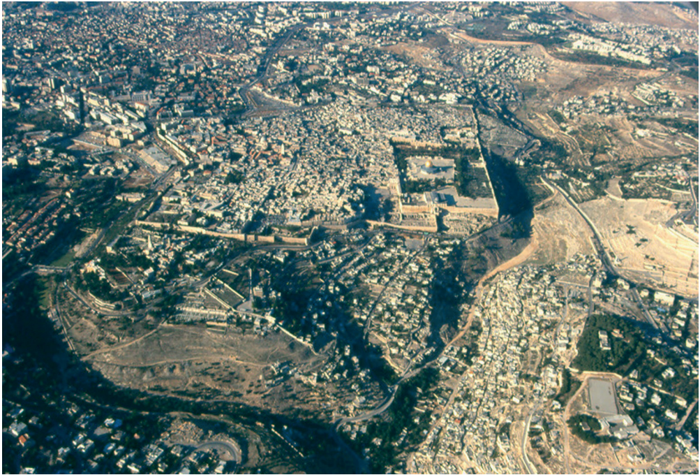
Fig. 2.1: Aerial view of the Old City from the south (G. Avni and the Israel Antiquities Authority).
