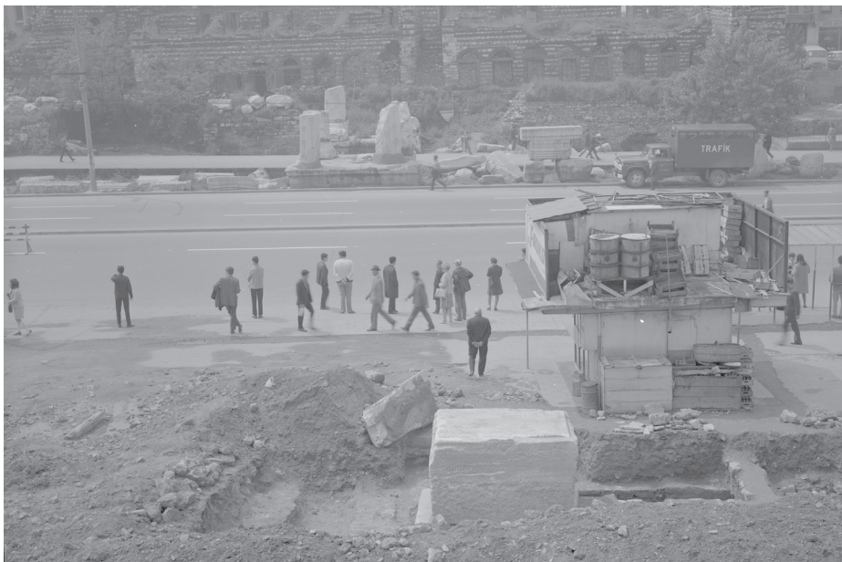
Fig. 7.1: Remains of one gate of the Forum of Theodosius, Beyazit, Istanbul, as exposed in 1969. Deutsches Archäologisches Institut Negative No. D-DAI-IST-69-3 (W. Schiele).
